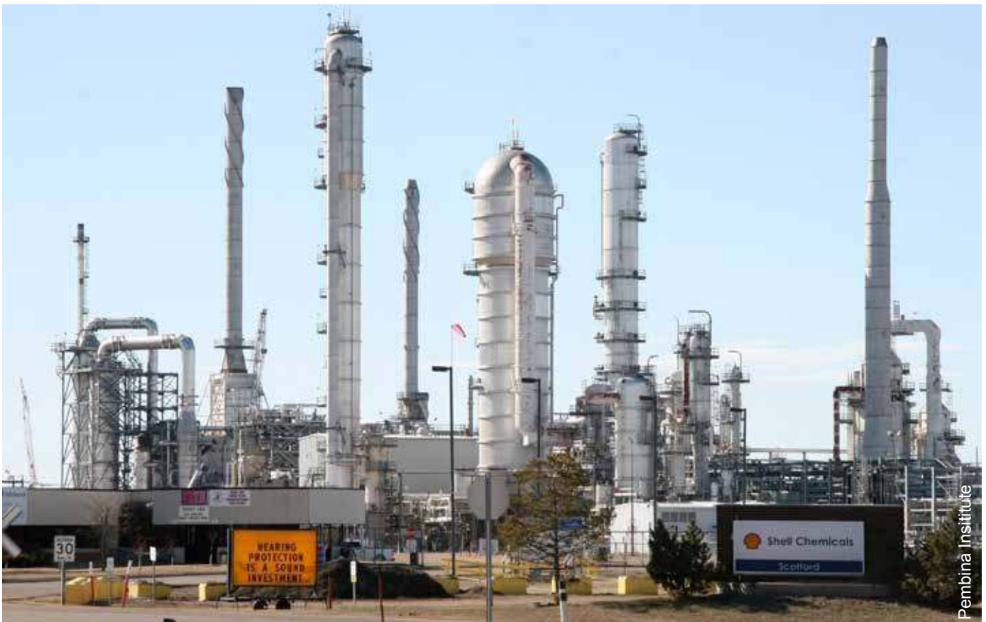
Shell's Scotford upgrader, which processes crude bitumen into a range of synthetic crude oils
