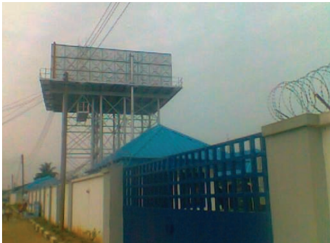
Eleme water supply system. Photo: Onyekachi Okoro Emmanuel
